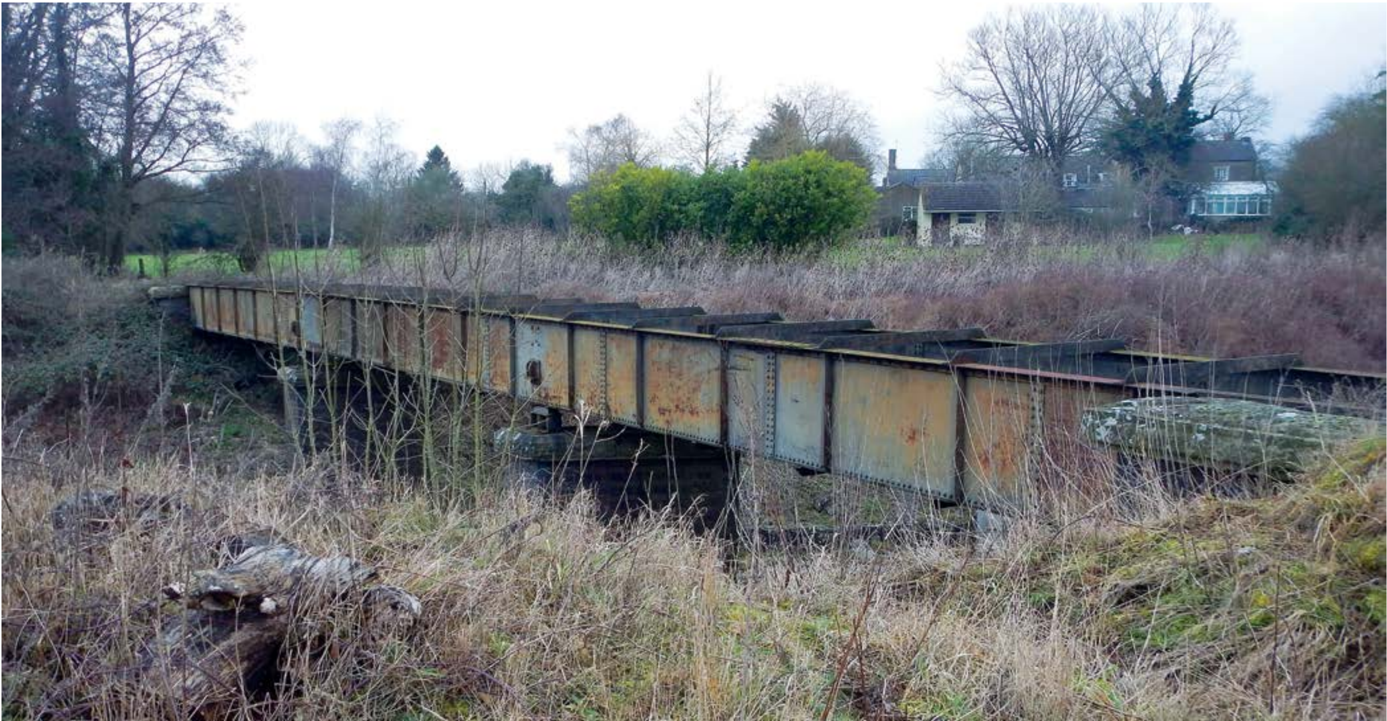
Ecosystem-based solutions can add value and produce diverse co-benefits in most policy settings, for example as a more sustainable option than this box channel carrying a river over a flood-prone railway cutting.
